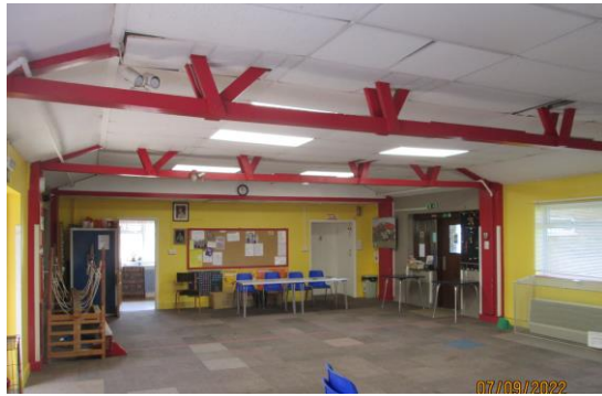
Photo 25 – View of main hall with exposed timber trusses
