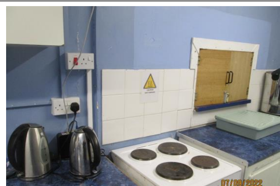
Photo 42 - Cooking area with cooker point and sockets close to oven and hob
